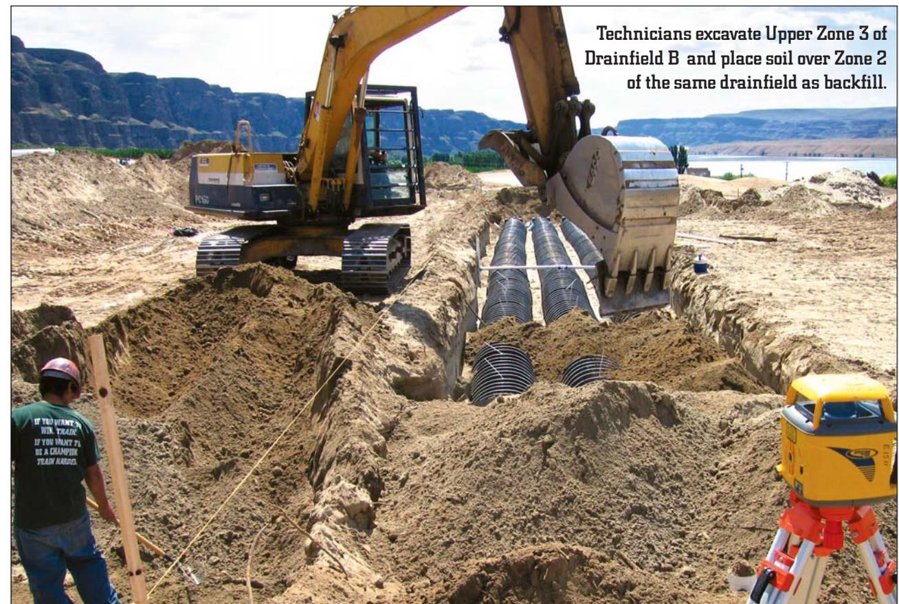
Technicians excavate Upper Zone 3 of Drainfield B and place soil over Zone 2 of the same drainfield as backfill.
