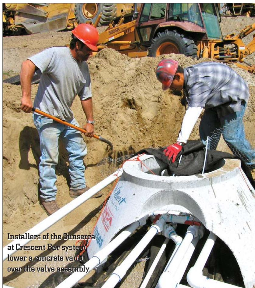
Installers of the Sunserra at Crescent Bar system lower a concrete vault over the valve assembly.
