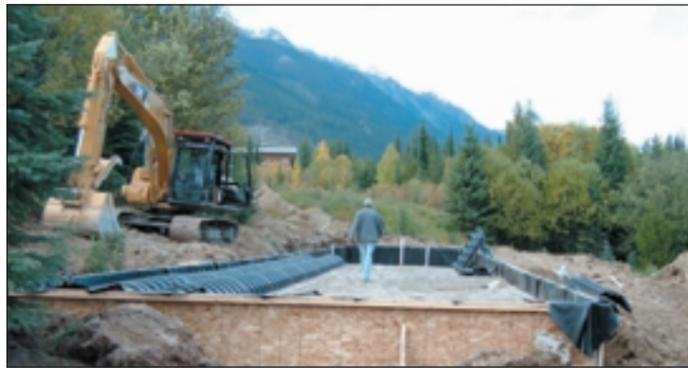
A sand filter nears final construction as the Infiltrator chambers are placed on the filter material. The chambers allow a better effluent dispersal and gas exchange.
