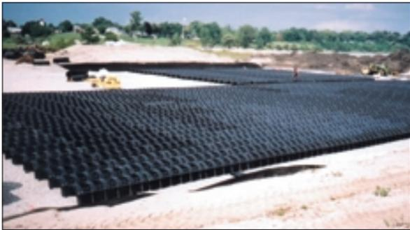
The exfiltration gallery at the Port Burwell Sewage Treatment Plant in Bayham, Ontario includes approximately 220 metres of Infiltrator High Capacity H-20 chambers. The construction of the bed includes 300 mm of clear stone as a base.
