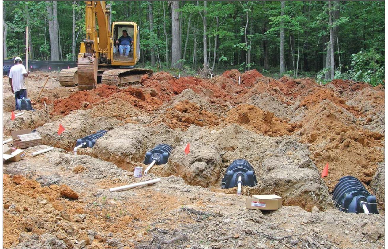
air. Wastewater enters the mixing tank and is oxygenated for 24 hours. This process produces the minimum of sludge and can handle widely varying hydraulic and biological flows. The mixed liquid then enters the clarifier from the bottom.
