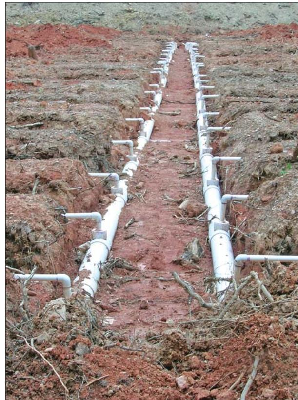
Above, 1,800 EQ36 chambers are installed in two-foot-wide trenches in the second section of the drainfield. At the left, two 6-inch lines carry effluent to the header line. Off the header line, the effluent travels through a tee, then to a distribution pipeline at the tops of the chambers.
