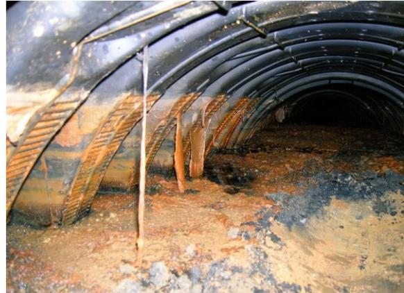
*Figure 2 - Drainfield inspection reveals paint in system*
