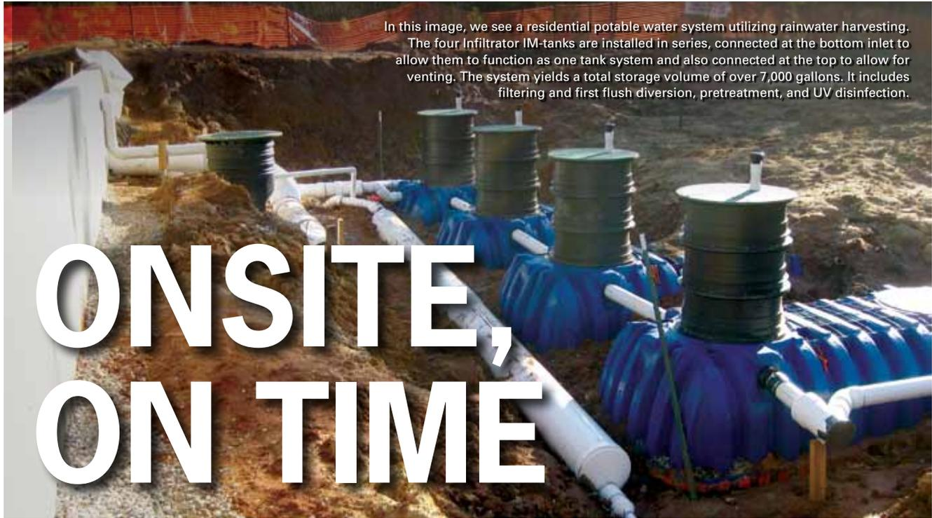
In this image, we see a residential potable water system utilizing rainwater harvesting. The four Infiltrator IM-tanks are installed in series, connected at the bottom inlet to allow them to function as one tank system and also connected at the top to allow for venting. The system yields a total storage volume of over 7,000 gallons. It includes filtering and first flush diversion, pretreatment, and UV disinfection.
