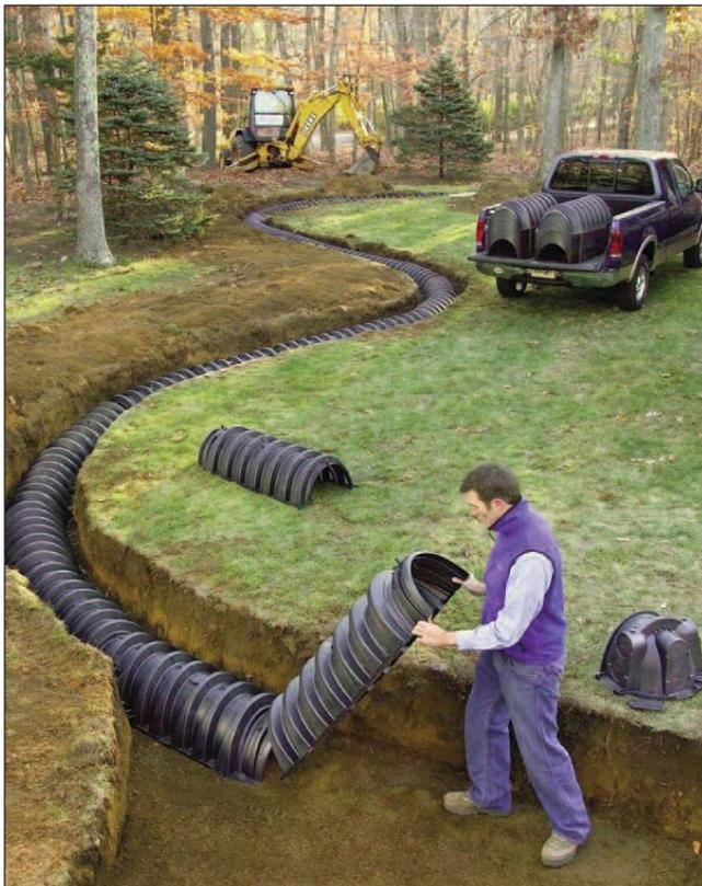
*Infiltrator chambers are the original plastic leachfield drainage chambers.*
